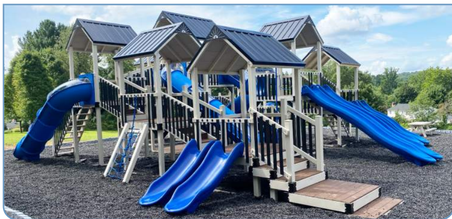
Our new playground area is well underway with more to follow!
